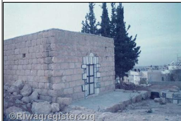
Figure 5.21: BaytUla village – house standing with Qassa in front of the apparent-framed door- small window in the side elevation without frame.
