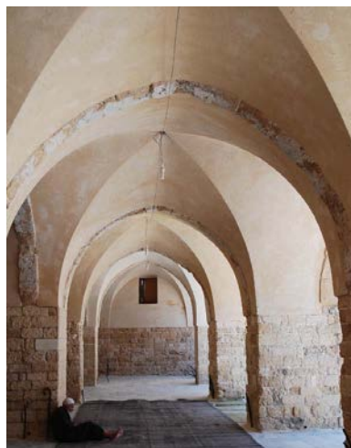
Figure 3.14: The vaulting construction of Omari Mosque in Gaza old city, Palestine. Source: Gaza Today.com, 2011
