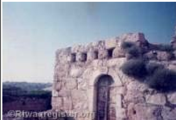
Figure 5.20: Hebron village house- the tiny openings of the dwelling
